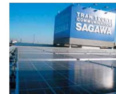
Solar power generation system
